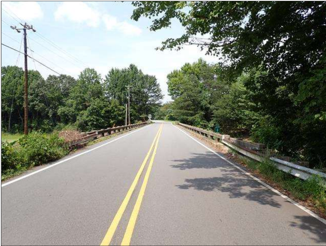
south approach looking north
