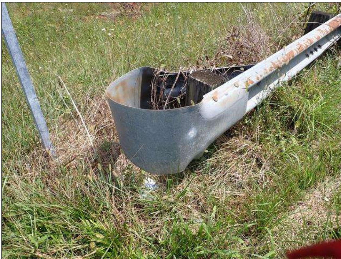
northeast guardrail termination
