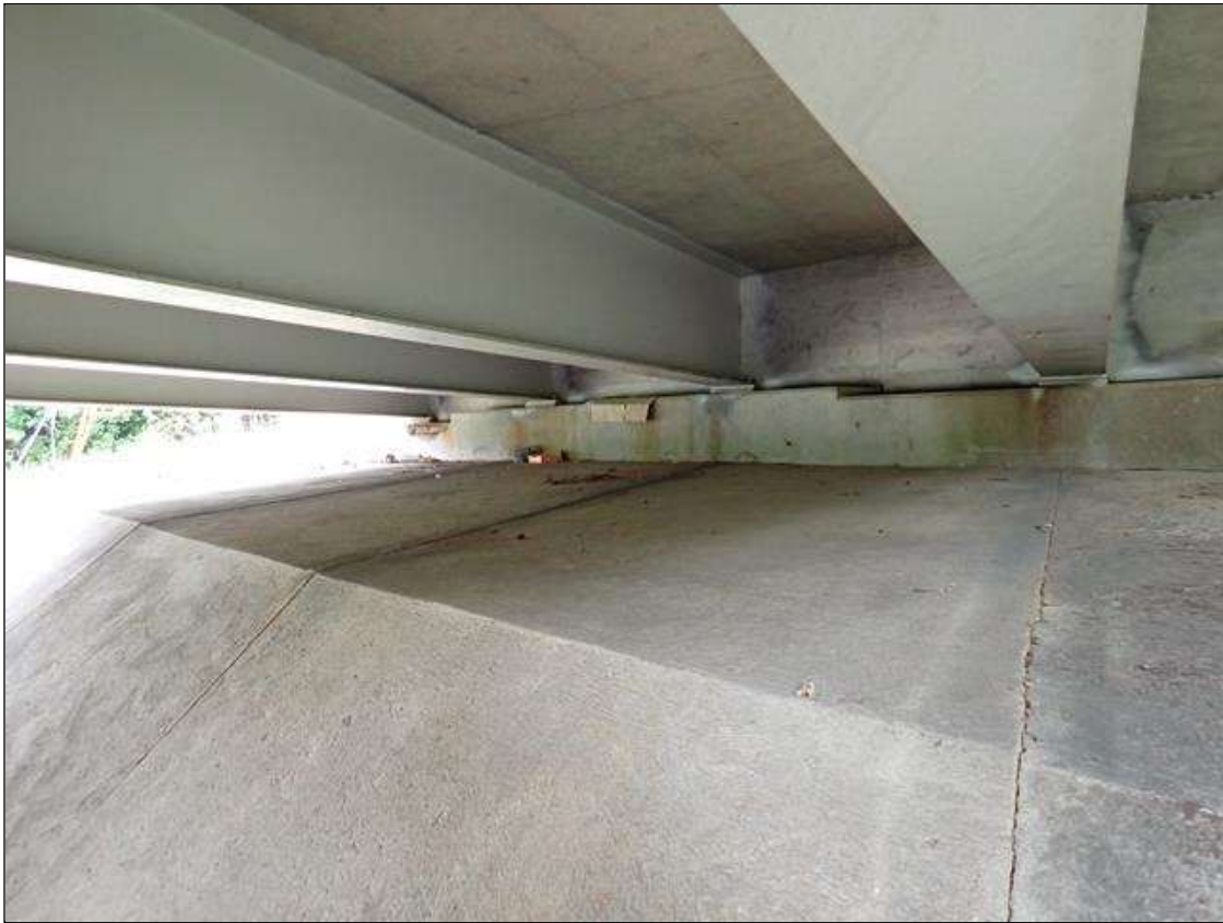
end bent 2 and slope protection
