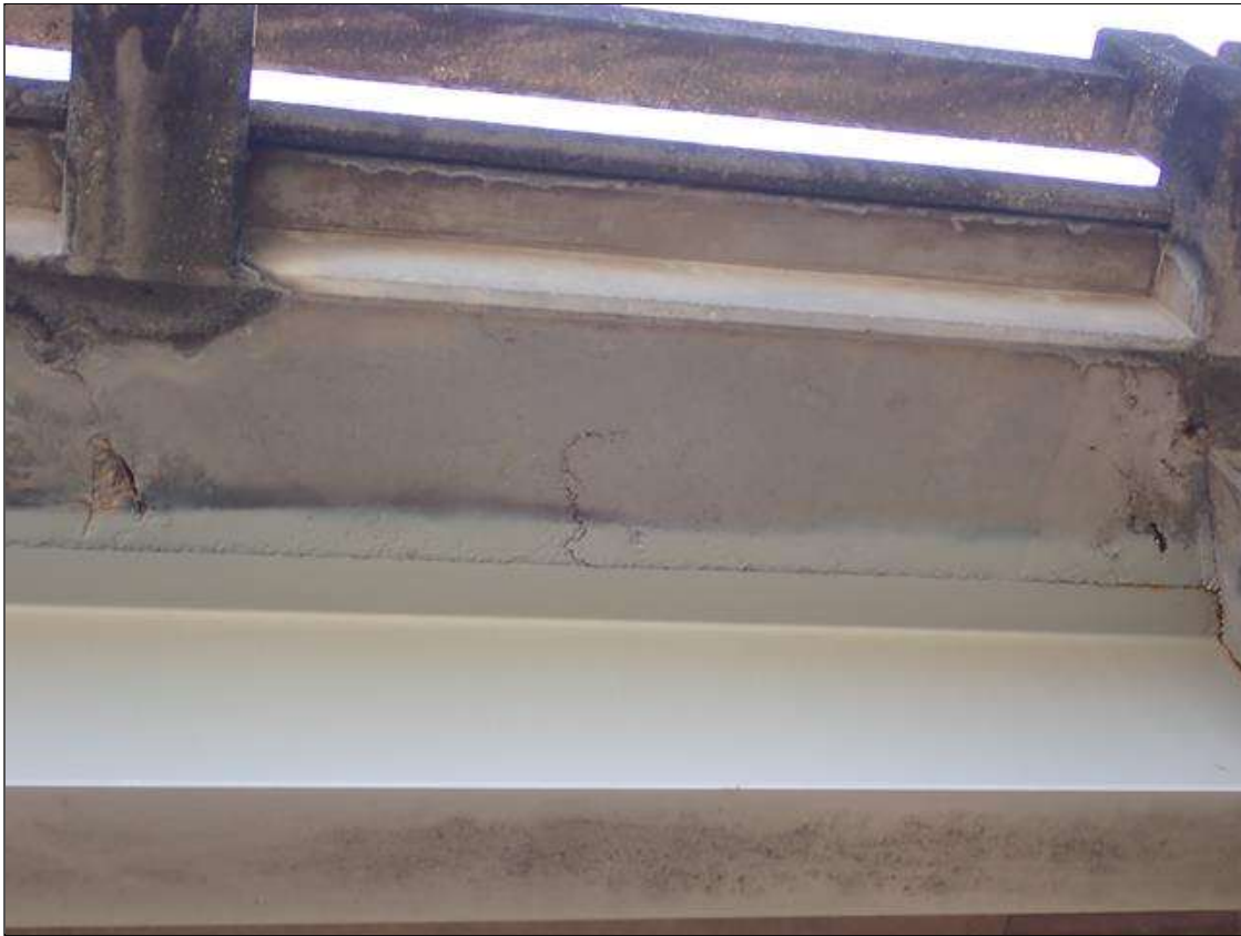
Span 3 Deck: (PAR) MULTIPLE UP TO 2 FOOT X 1 FOOT X 1 DEEP SPALL/DELAMINATION WITH EXPOSED REBAR AT RANDOM THROUGHOUT WEST OVERHANG; SOME DELAMINATION OVER TRAVEL LANES
