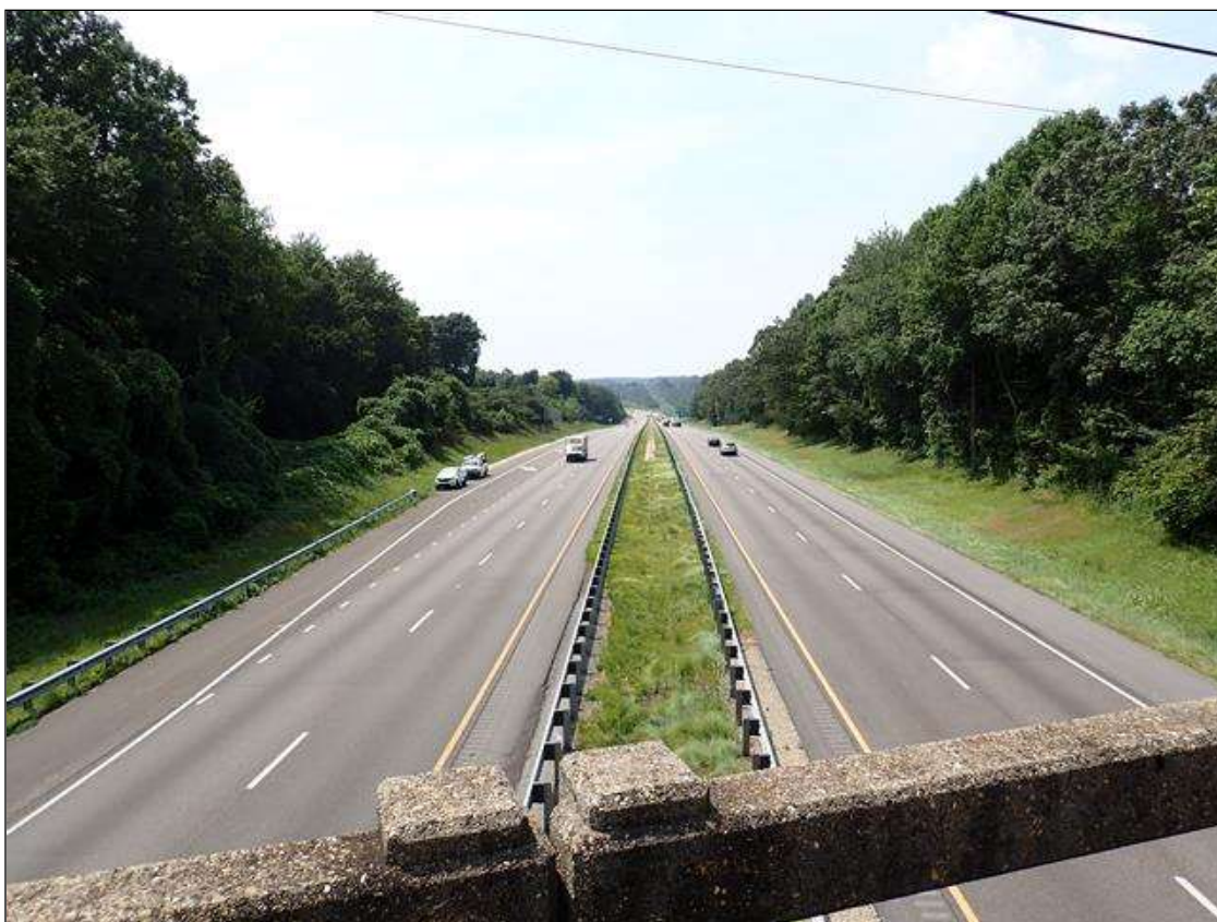
roadway looking west
