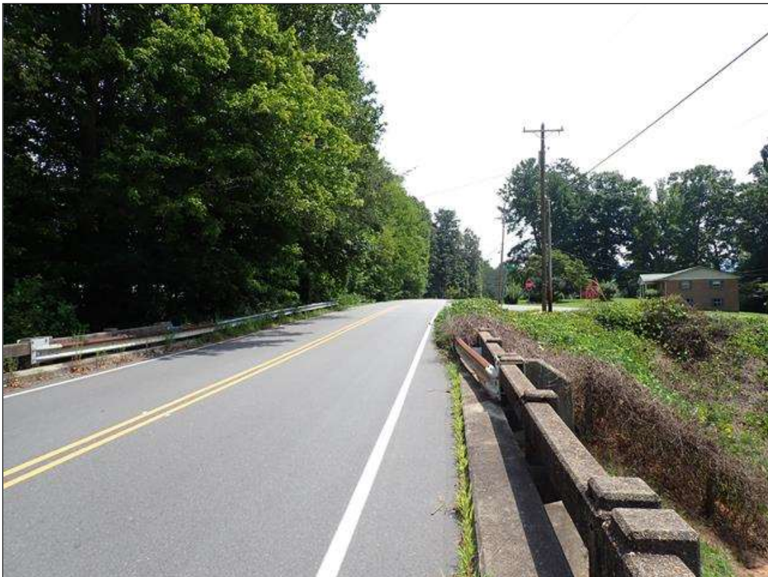
south approach looking south
