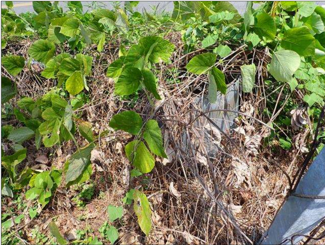
southwest guardrail termination
