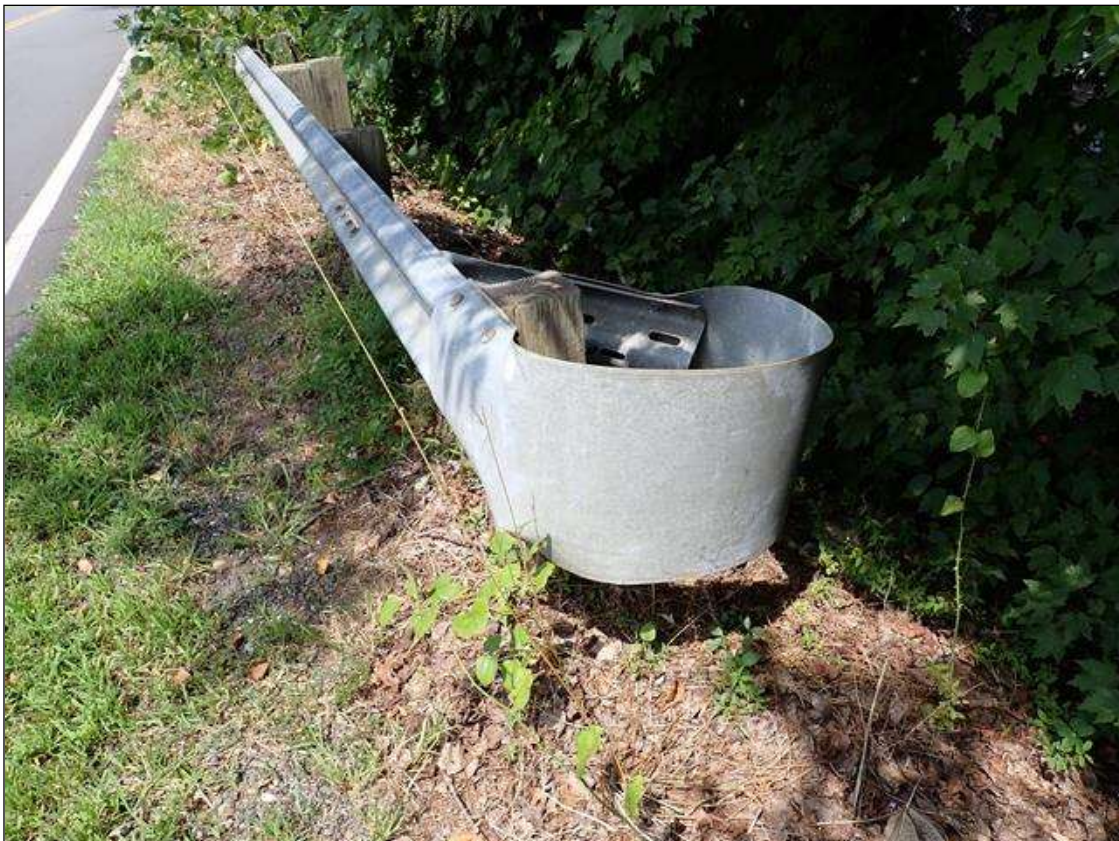
southeast guardrail termination
