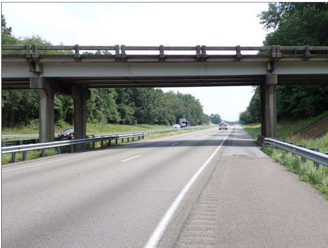
roadway under span 2, looking east (I-40 eastbound)
