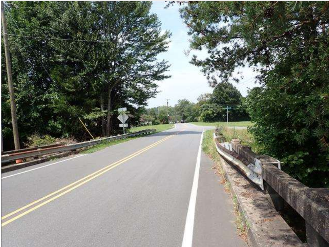
north approach looking north
