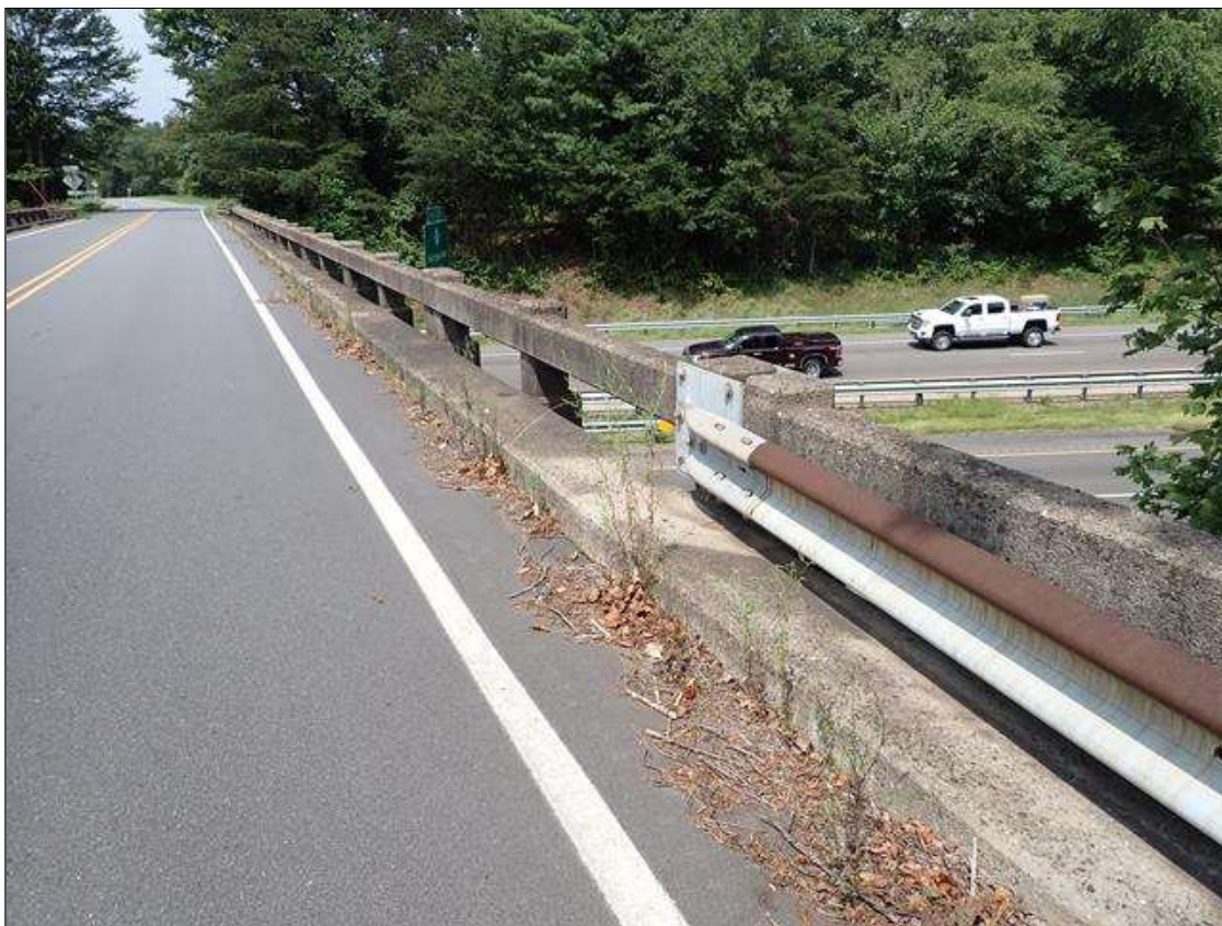
right bridge rail
