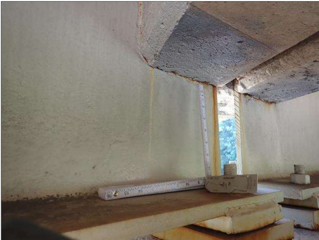
Span 3 Beam 4: at bent 2, corrosion with section loss: web adjacent to end diaphragm (9/16 inch average remaining x 10 inch x 1 inch)
