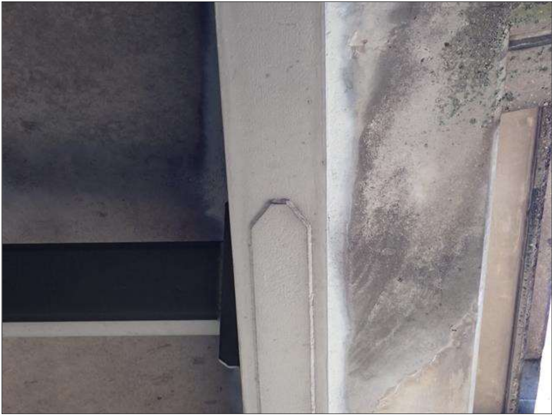
typical cover plate termination
