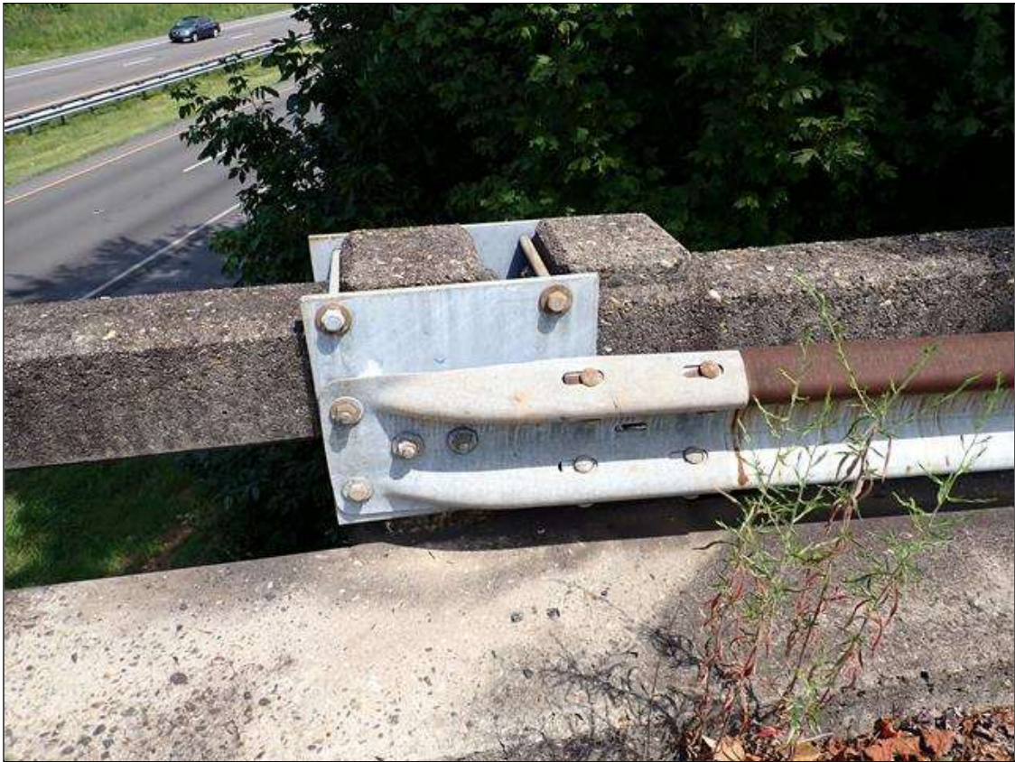
southeast guardrail attachment
