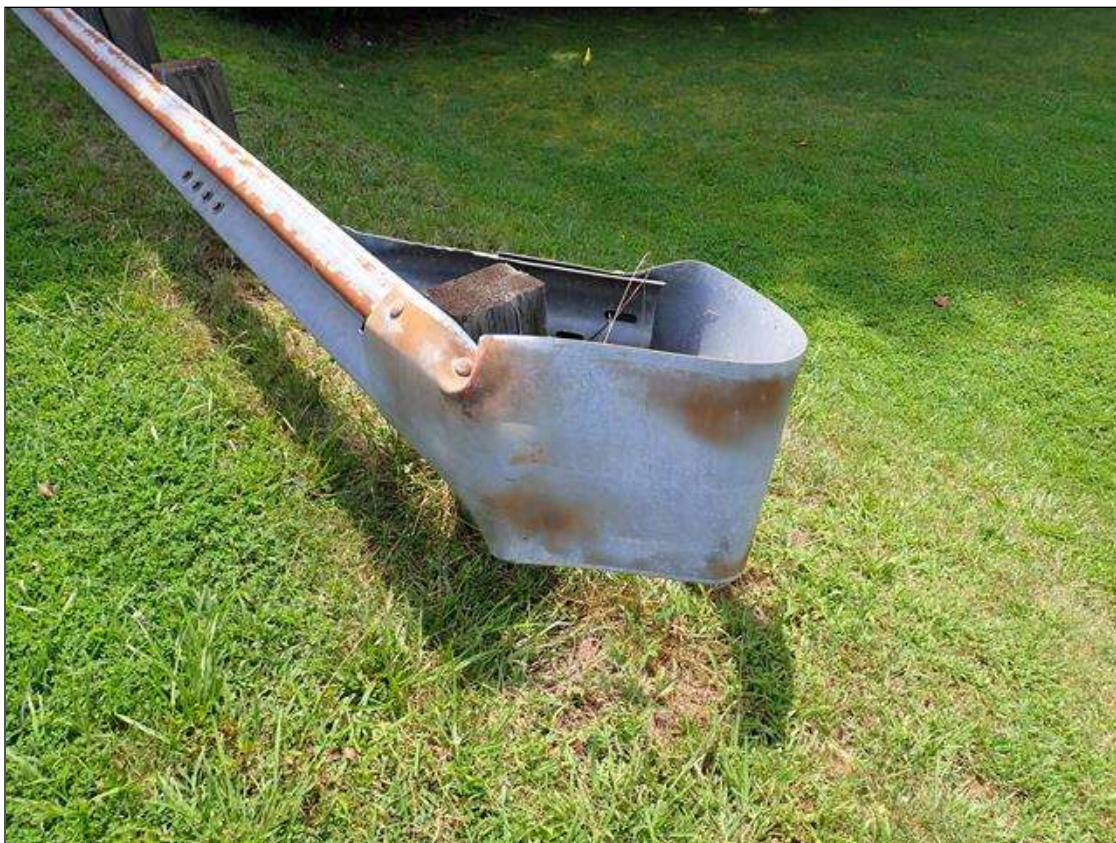
northwest guardrail termination
