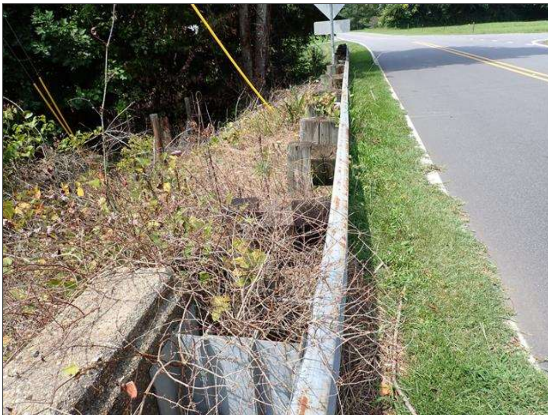
northwest guardrail transition
