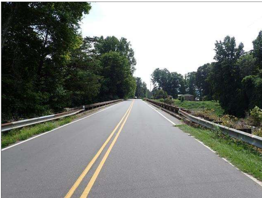
north approach looking south
