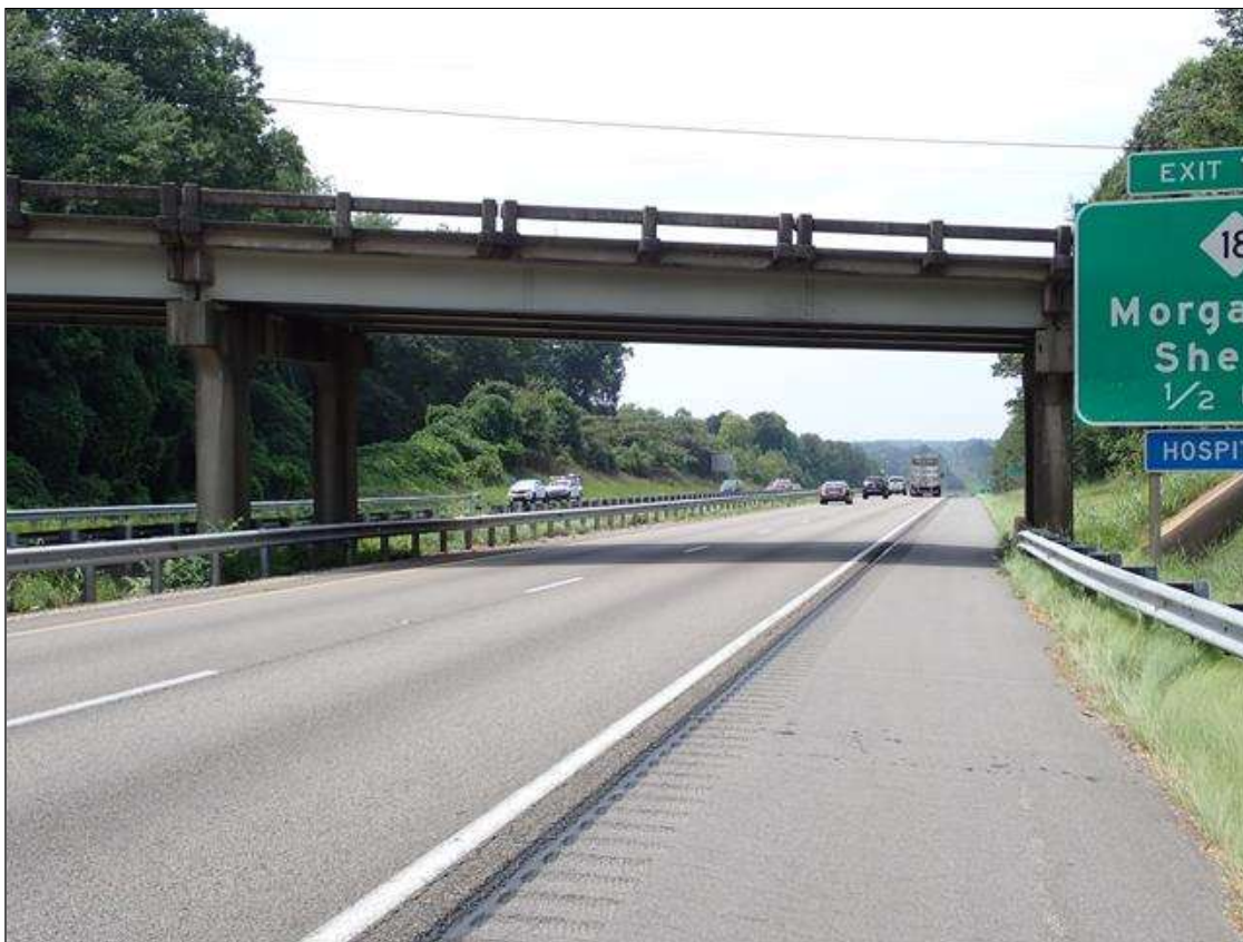
roadway under span 3, looking west (I-40 westbound)
