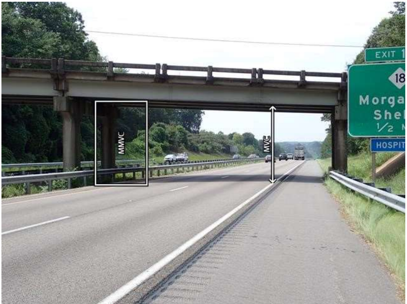
roadway under span 3, looking west
