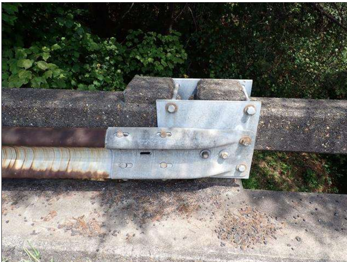
northeast guardrail attachment
