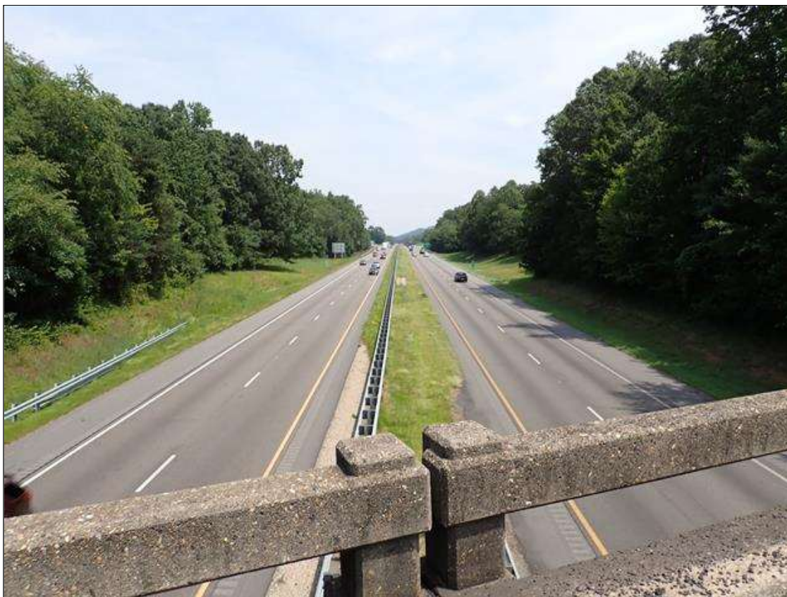
roadway looking east
