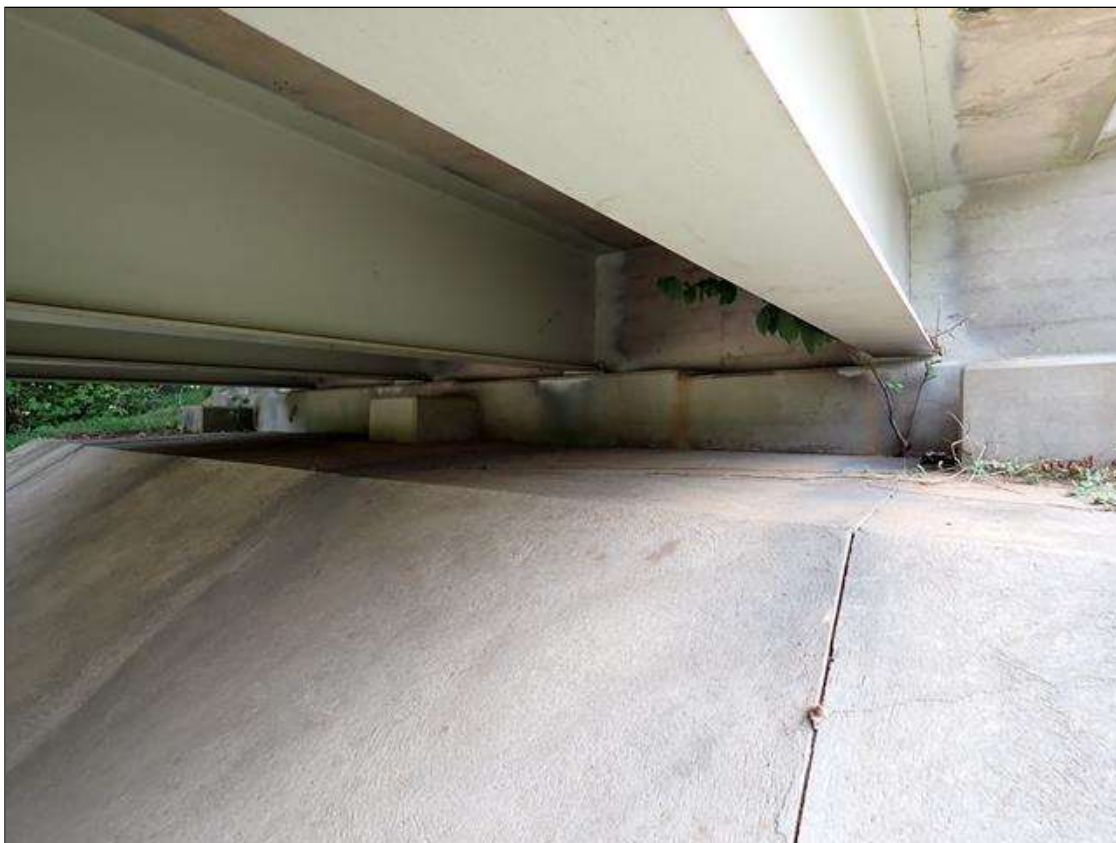
end bent 1 and slope protection
