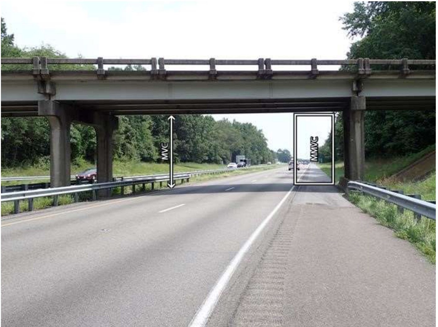
roadway under span 2, looking east
