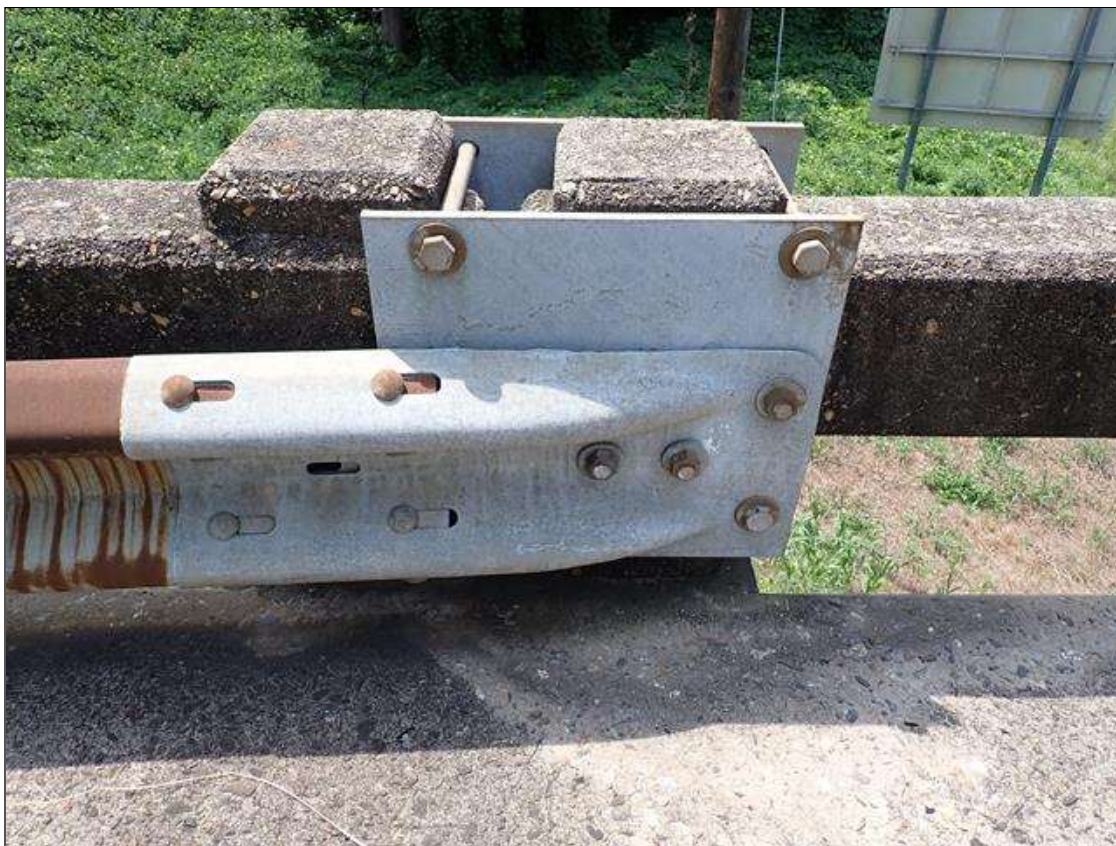
southwest guardrail attachment
