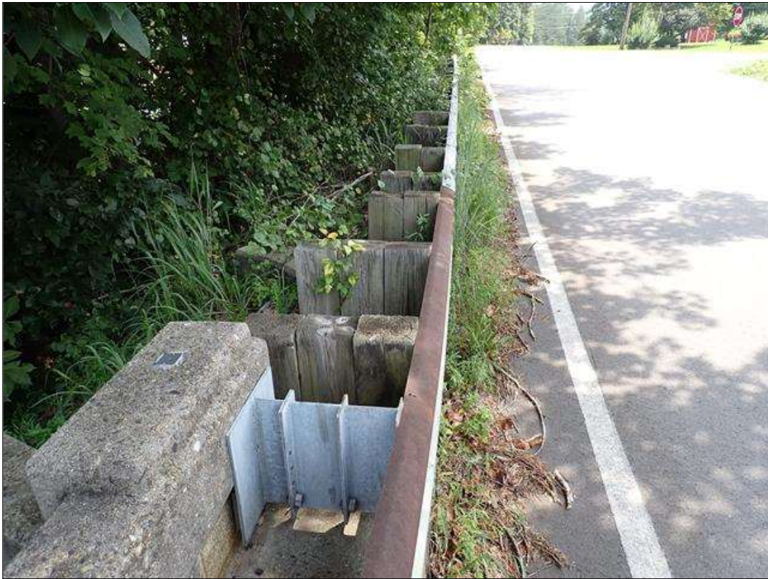
southeast guardrail transition
